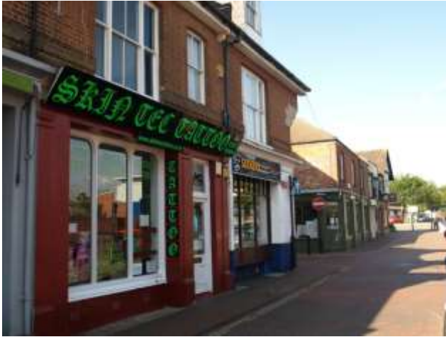
New Street (left) has a domestic scale of generally 2 storey properties with restrained shop fronts. A gable ended building acts as a 'book end' to this part of the street. Some over-large fascias intrude into the character of the building and street scene.
