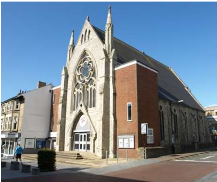
Despite the unfortunate flat roofed brick side extensions and the slight recess from the general street frontages, the contrasting scale, use of ragstone (reminiscent of St Mary's church) and prominent location set above steps at the centre of Bank Street within a wide paved apron, Centrepiece Church is a prominent notable local building.
